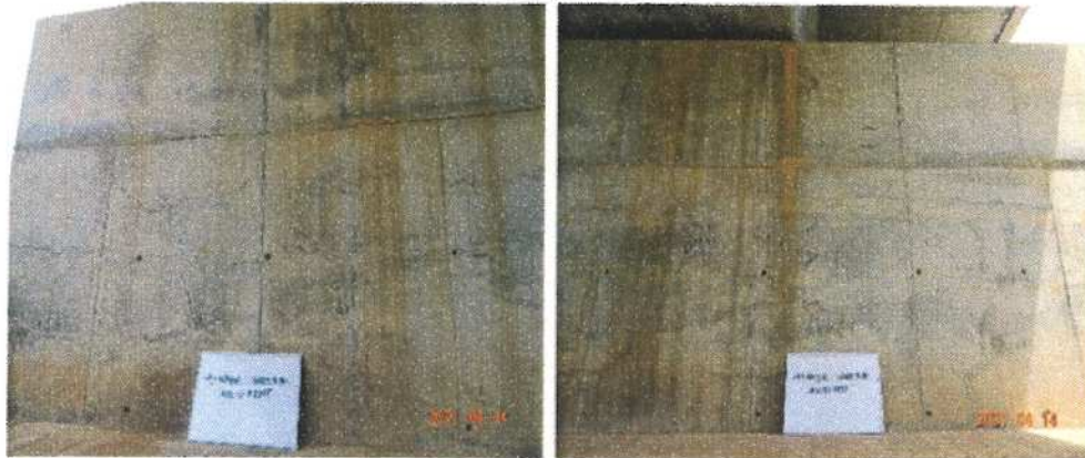
A1 abutment front
