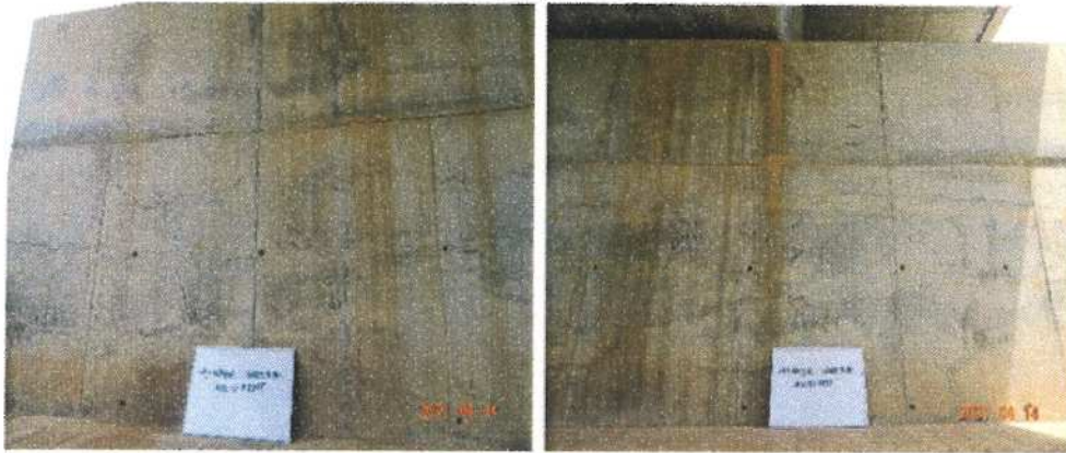
A1 abutment front
