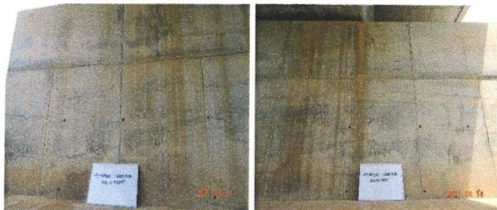
A1 abutment front
