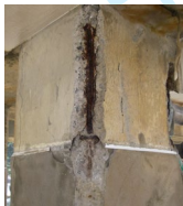
Photo2 Reinforcing bar part of C1
