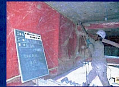
⑤圧入孔削孔
