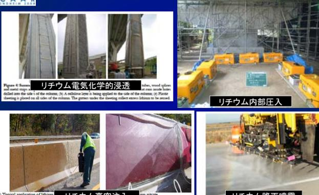
Figure 4 Summary: リチウム電気化学的浸透 (lithium, wood preservatives, etc. can be applied to the side of the column. A redstone time is being applied to the side of the column. Plastic sheeting is placed on all sides of the column. The gaskets under the sheeting collect excess lithium to be reused.)
