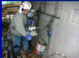
⑤圧入孔削孔
