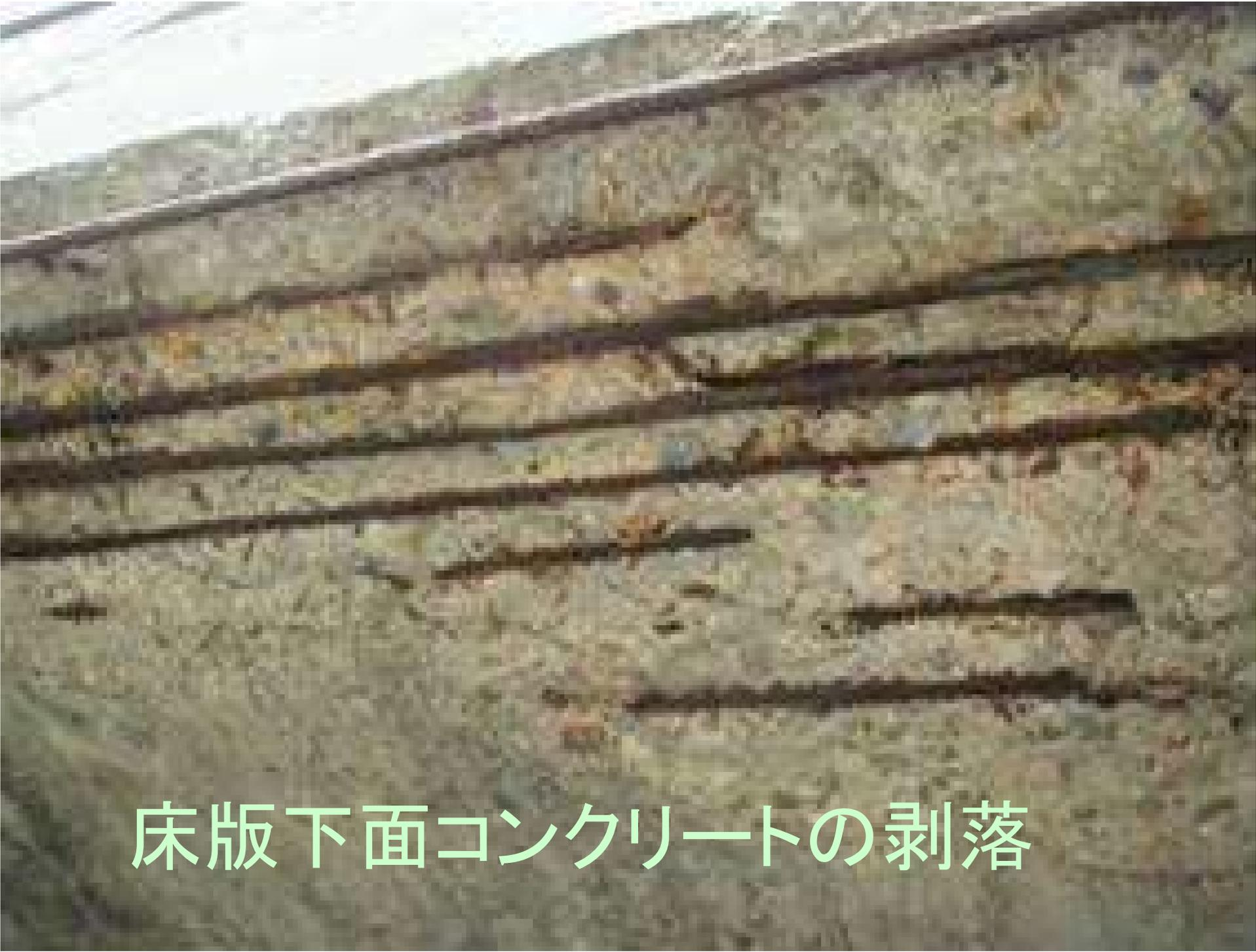
A photograph showing the underside of a bed board. The concrete surface is heavily damaged, with large areas of peeling and crumbling. The remaining concrete is dark and uneven, with visible layers and textures. The background is a plain, light-colored wall.
