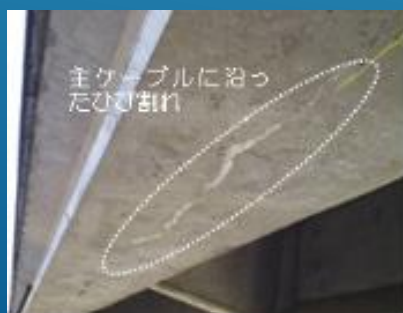
PCT 桁下面に発生したひび割れ事例 (Example of cracks occurring on the underside of the PCT truss)
