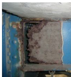
H21損傷状況 (主桁腐食)
