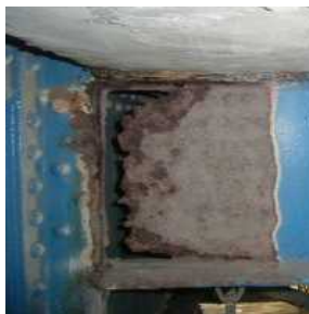
H21損傷状況 (主桁腐食)
