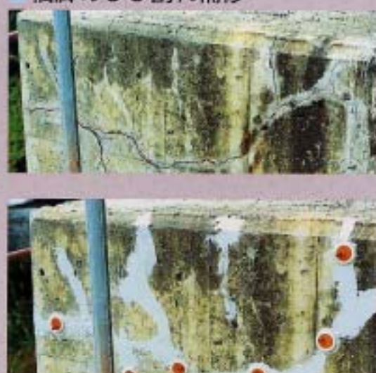
● 橋脚のひび割れ補修
