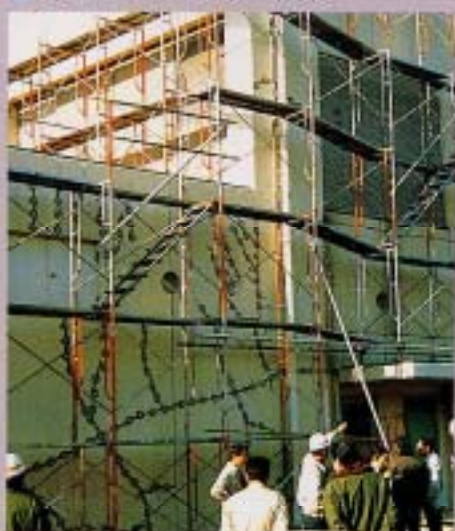
● 外壁のひび割れ補修
